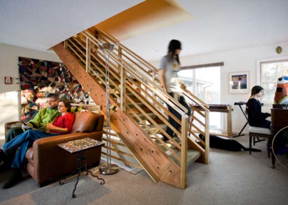
Louise Robinson and Neal Cuthbert's GreenStar-certified remodeling project included the construction of a stairway from rafters they removed during the addition of a second story. The family worked with many local professionals to save and reuse all the wood taken off the house before the new construction started.
