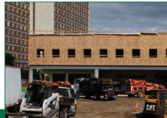
Construction of the addition started in early April 2008.
