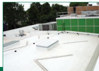
White roofing conserves energy and minimizes heat-island effect.
